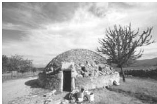
Figure 9. Cistern in Bodrum ( http://www.bodrubaglari.com/Yoremiz.html )
